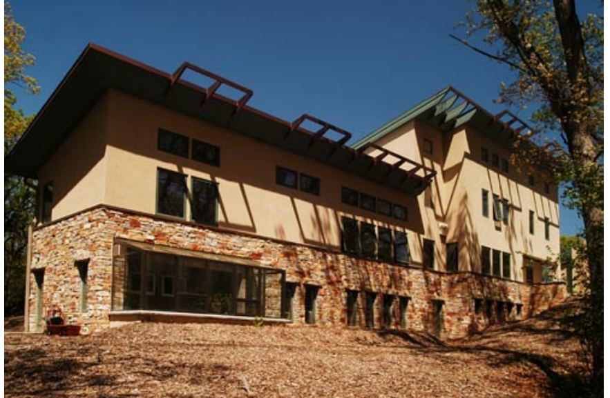
Limestone from a local quarry accentuates the south elevation otherwise designed for solar energy.
